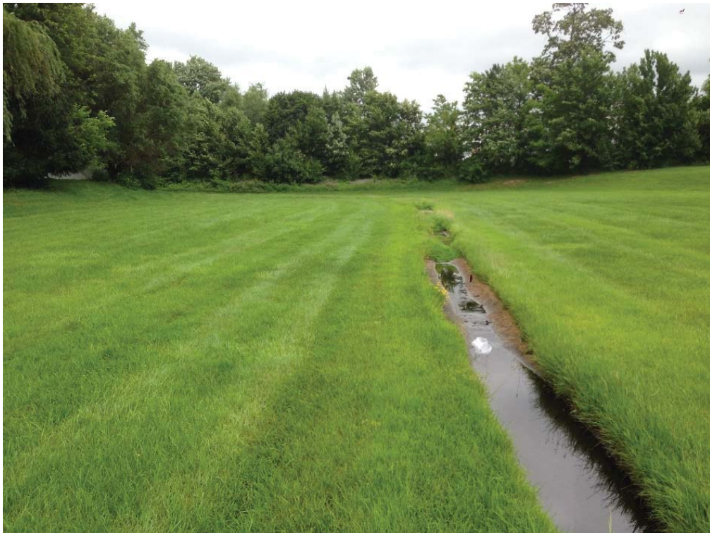
Photo 10 Proposed BMP-D: Cottonwood Court BMP Retrofit
