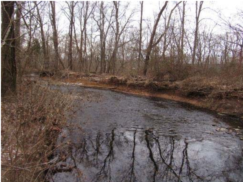
Photo 2- view looking downstream showing near vertical and eroding stream banks.
