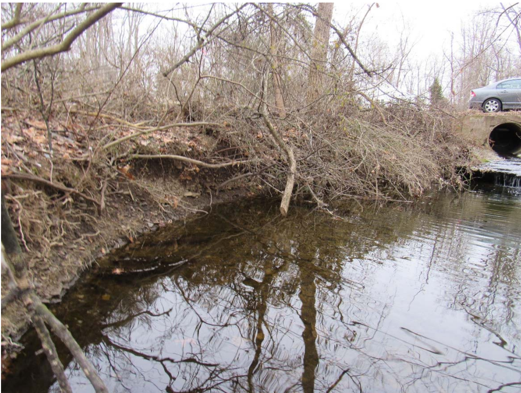
Photo 2 View looking upstream showing eroded stream bank and undermined concrete splash apron
