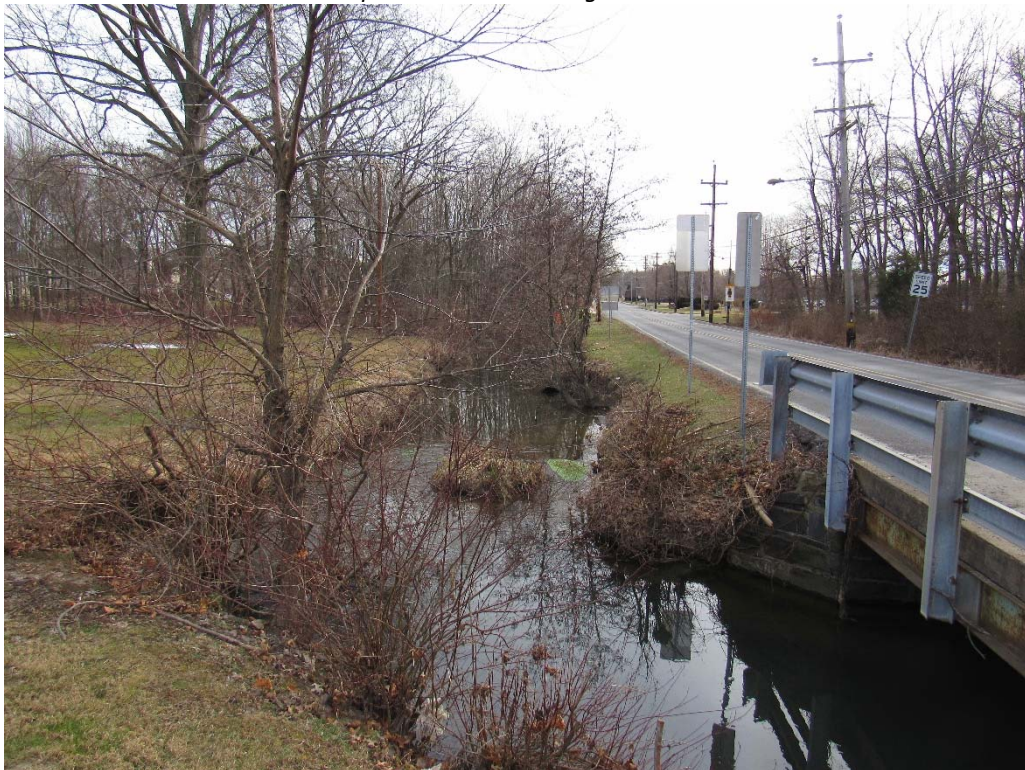
Photo 8 View looking upstream from Limekiln Road bridge. The area on the left side could be excavated to create a better floodplain connection. Limited opportunity exists for riparian zone enhancement along the south side of the channel due to required ROW restrictions
