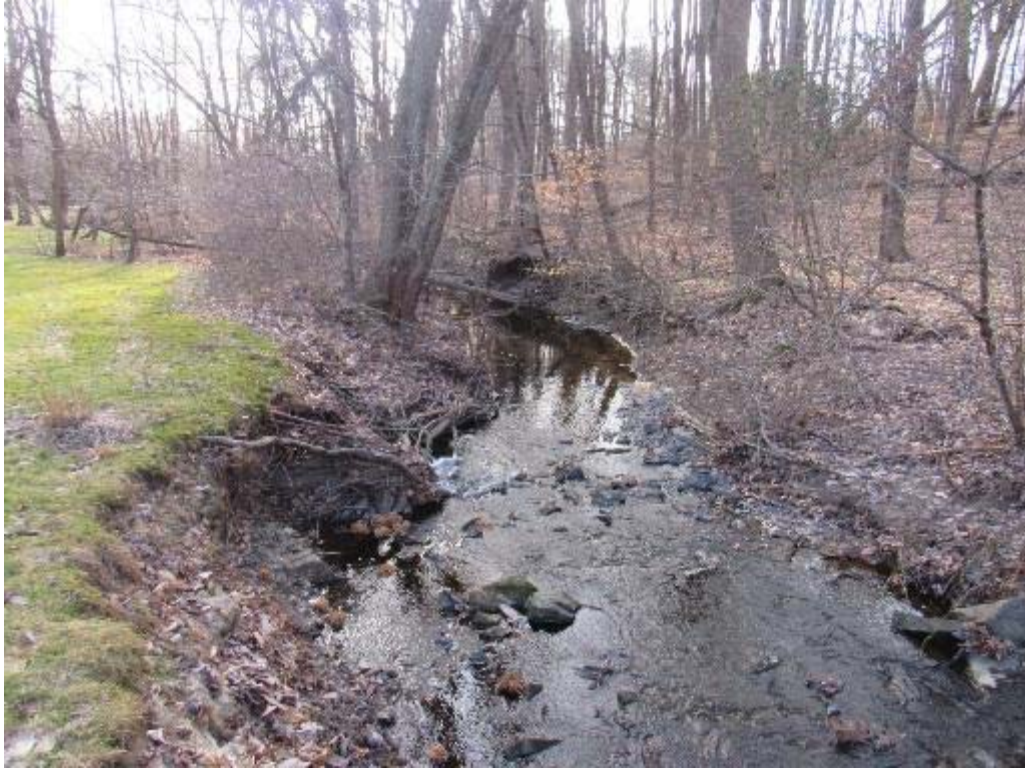
Photo 13 View looking downstream approximately 350 feet upstream of Turk Road. The channel is cut to bedrock with eroding stream banks and no floodplain access
