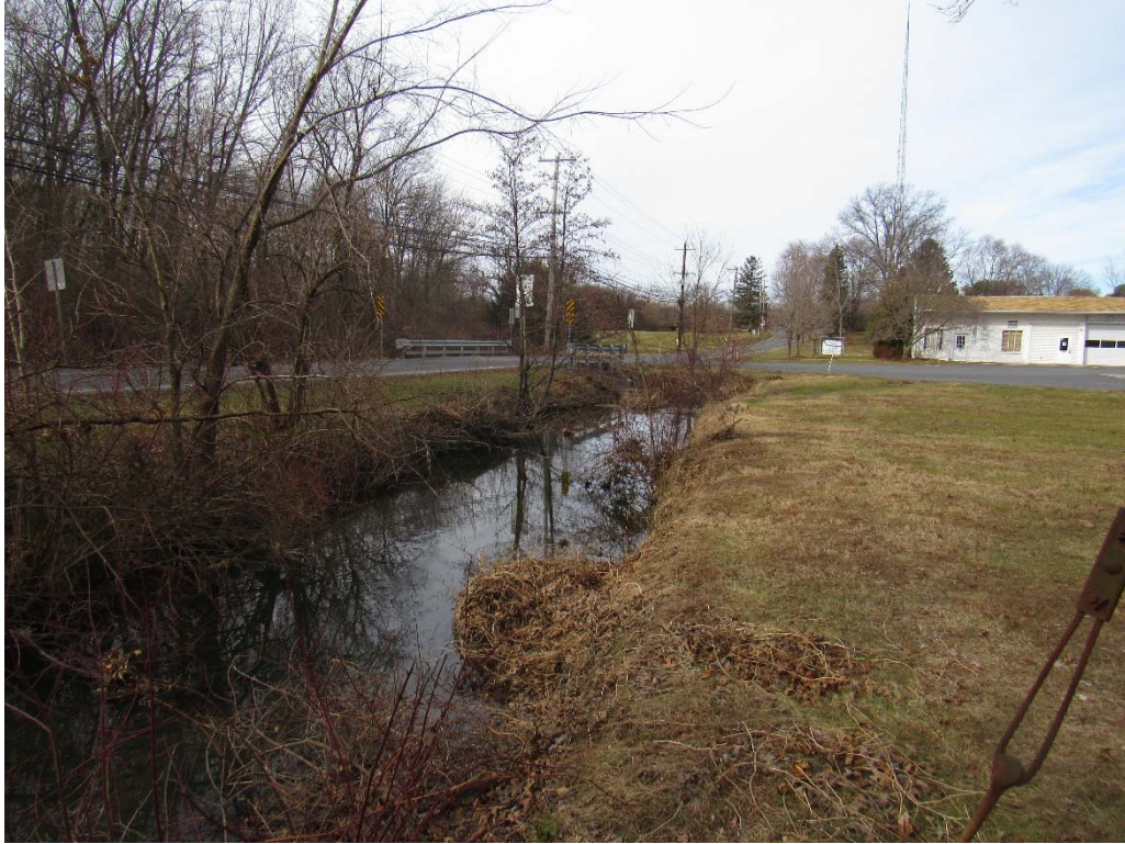
Photo 7 View looking downstream. The channel is entrenched with bank erosion along the left bank and a mowed riparian zone on the right bank.
