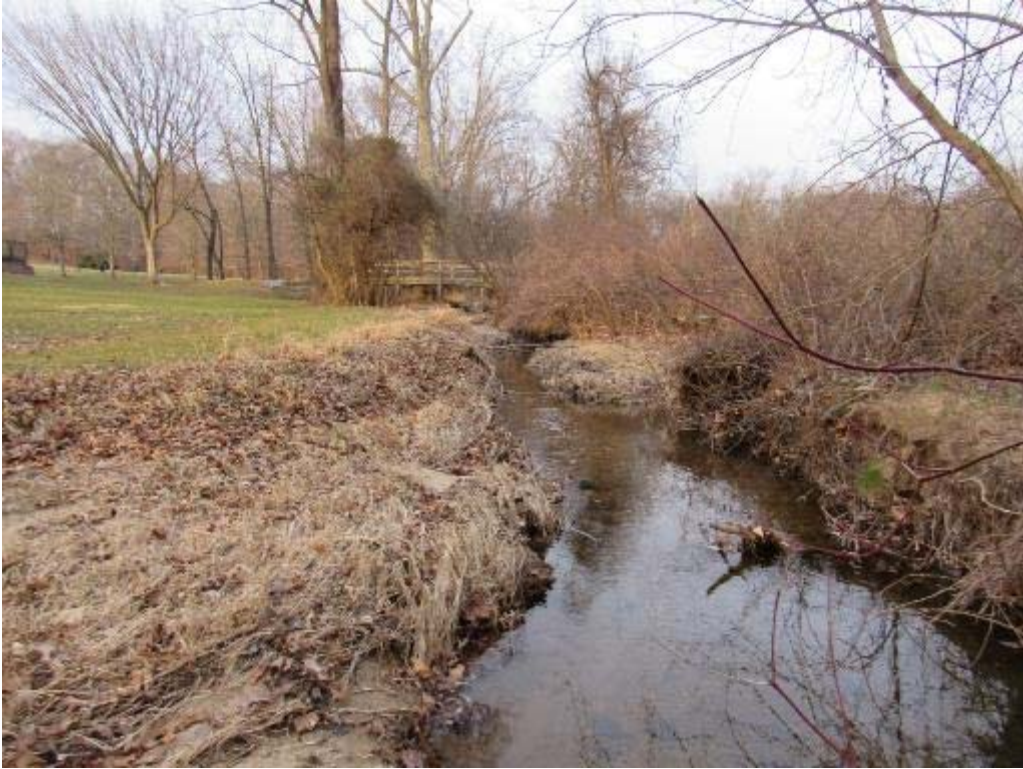
Photo 3 View looking upstream of Trail bridge crossing. Note vertical stream bank and erosion on the east bank and limited riparian vegetation.
