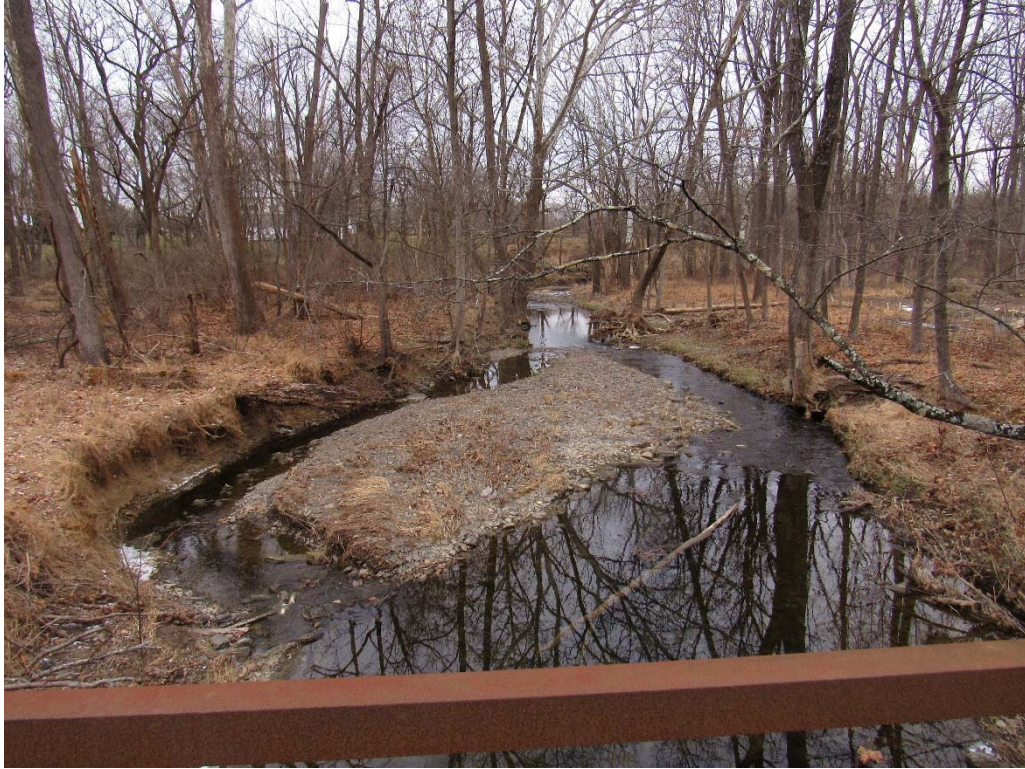
Photo 3 View looking downstream showing mid channel gravel bar development, channel widening and stream bank erosion
