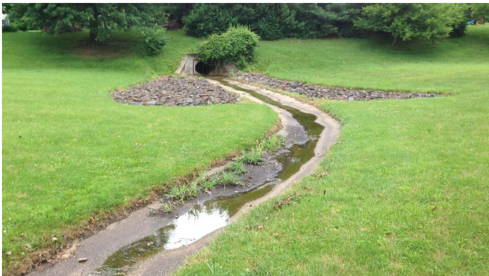
Photo 7 Proposed BMP-B: Ridings at Covered Bridge BMP Retrofits
