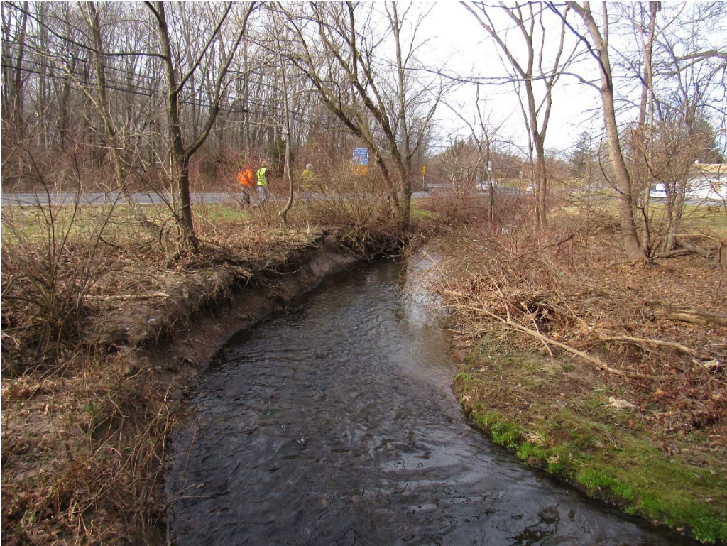
Photo 6 View looking downstream where Cooks run flow just north and parallel to Limekiln Road for 180 feet. Stream bank erosion is present along the south side of the channel.
