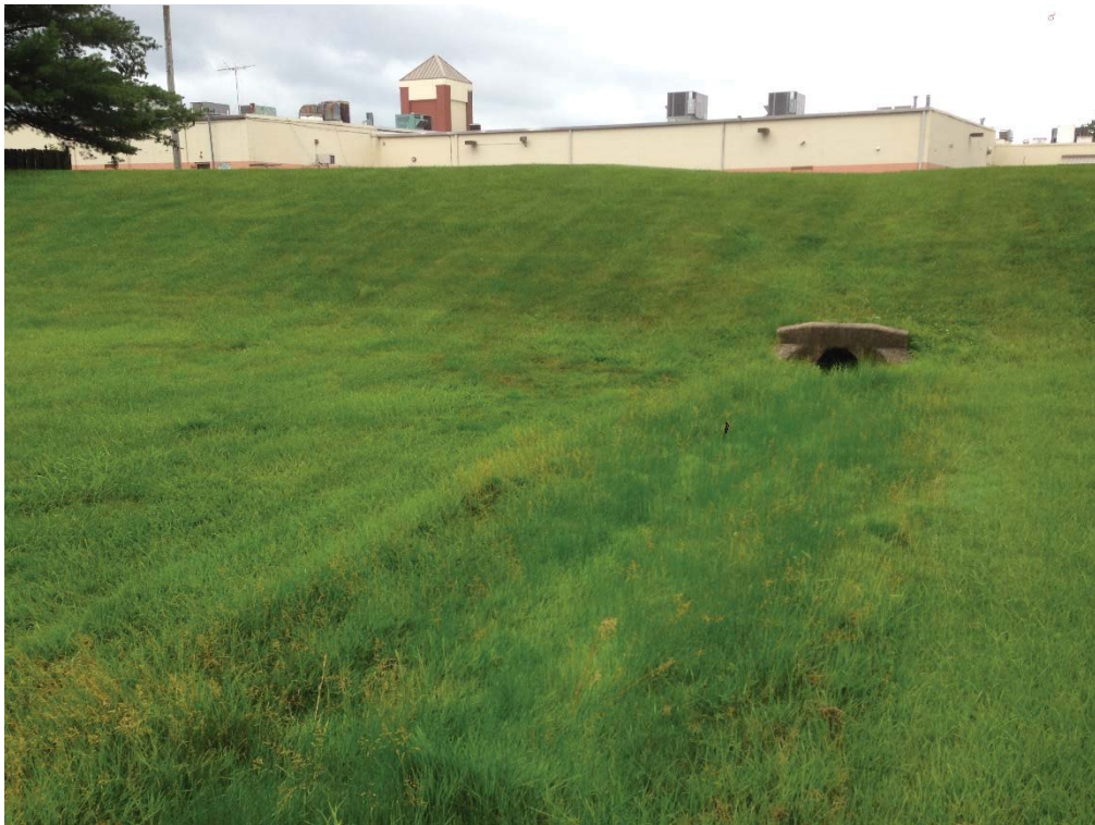
Photo 9 Proposed BMP-D: Cottonwood Court BMP Retrofit
