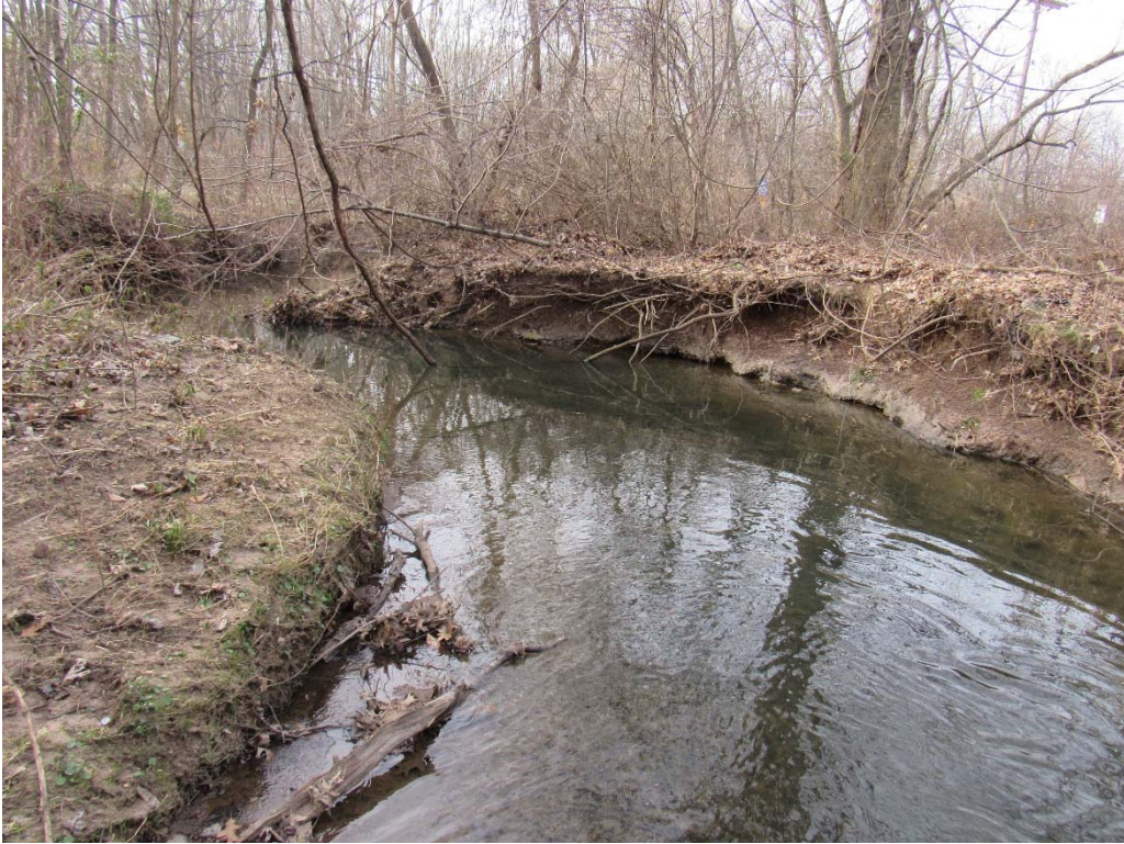
Photo 5 View looking downstream at eroded stream banks. There appears to be some limited connection to floodplain along the reach.
