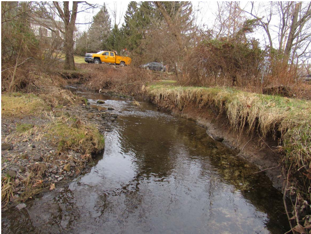
Photo 2 View looking upstream at eroding stream bank. The stream is slightly entrenched and could benefit from minor channel adjustments to provide better floodplain connection.
