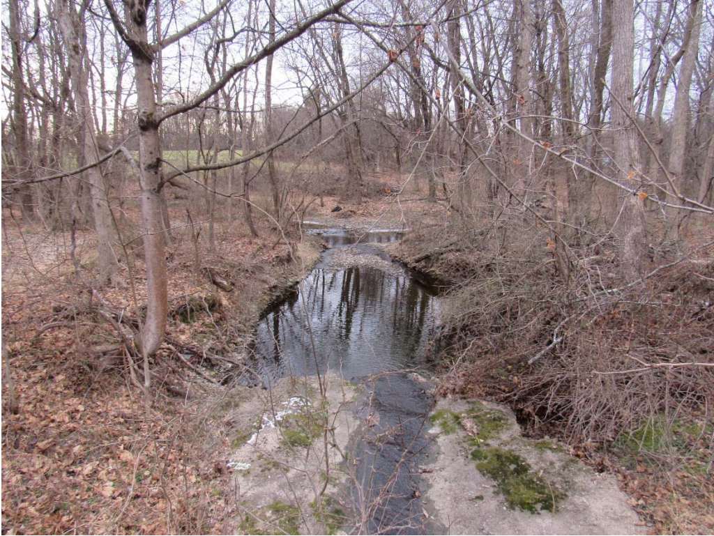
Photo 1 View looking downstream at eroded stream banks
