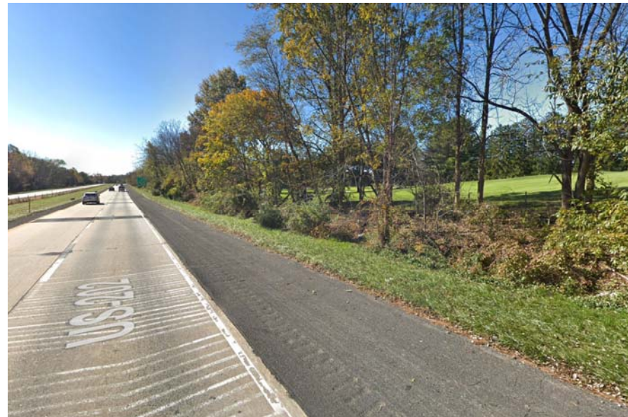
Existing New Britain Rd bridge over 611 Bypass (top) and Route 202 southbound with Doylestown Country Club golf course on right of photo (bottom).
