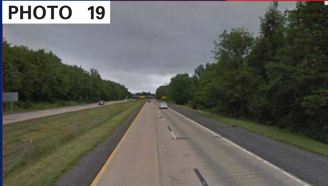
LOOKING NORTHBOUND ALONG 202 NORTH
