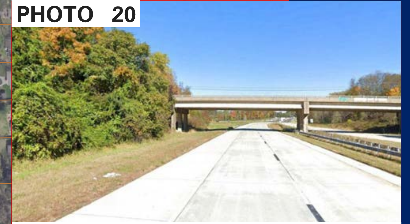
LOOKING NORTHBOUND ALONG 202 SOUTH TOWARDS EAST ROAD BRIDGE
