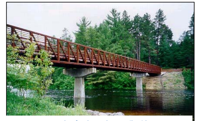
Example of Independent Trail Bridge
