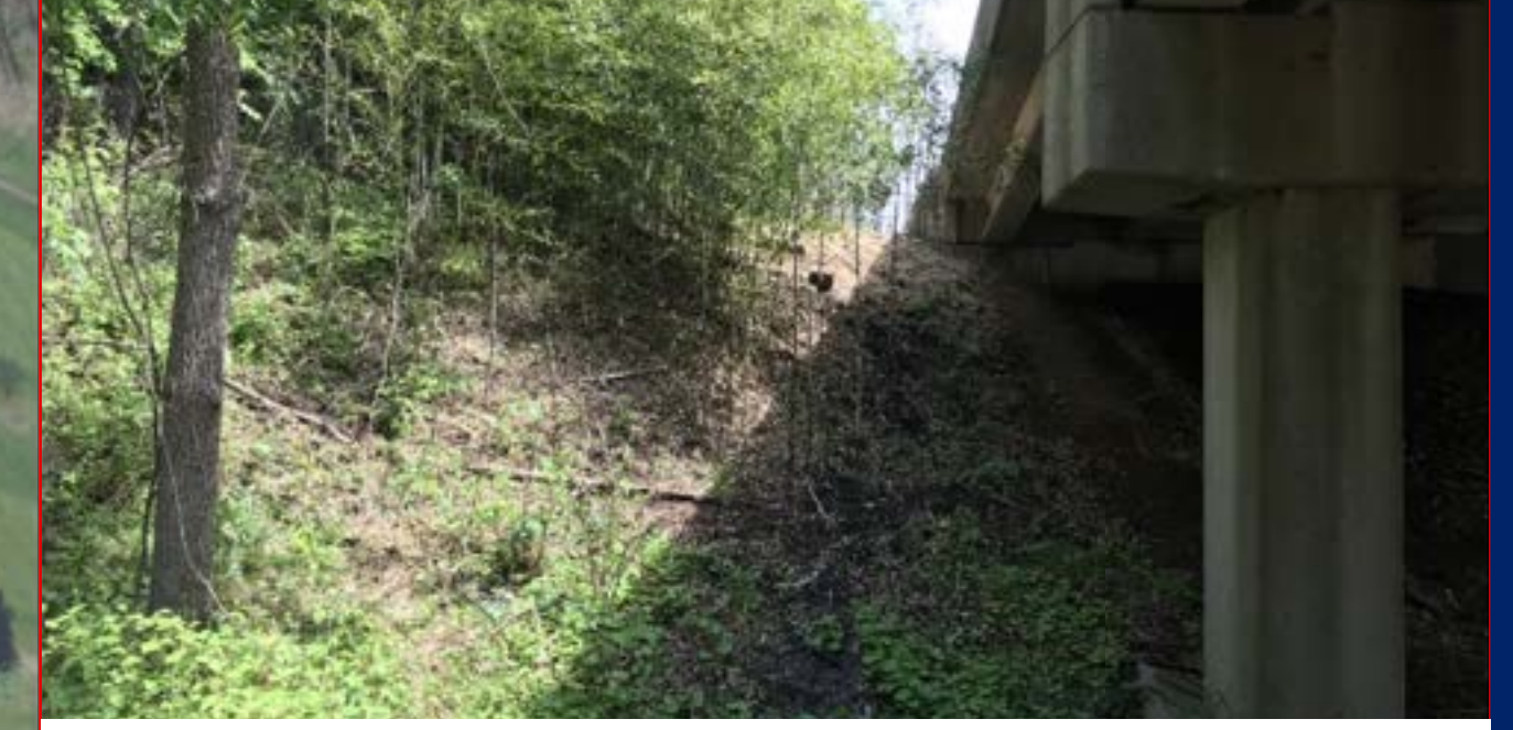
LOOKING FROM PEBBLE HILL ROAD/GREEN STREET NORTH
