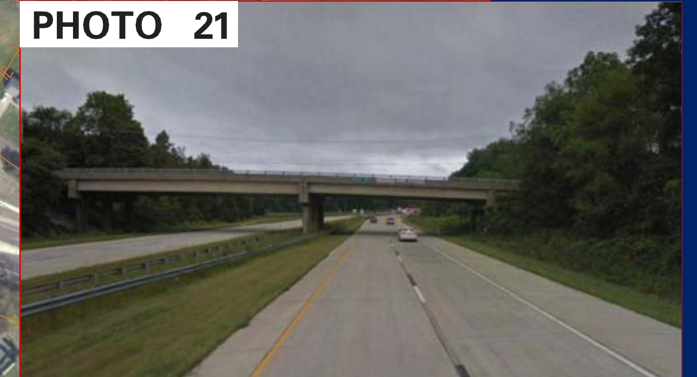
LOOKING NORTHBOUND ALONG 202 NORTH TOWARDS EAST ROAD BRIDGE
