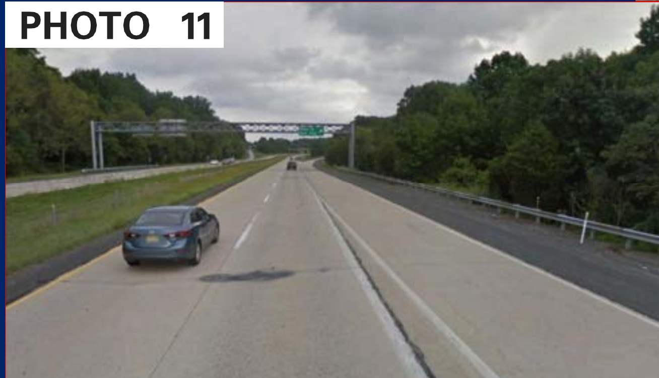
LOOKING NORTHEAST ALONG 202 OFF RAMP 2
