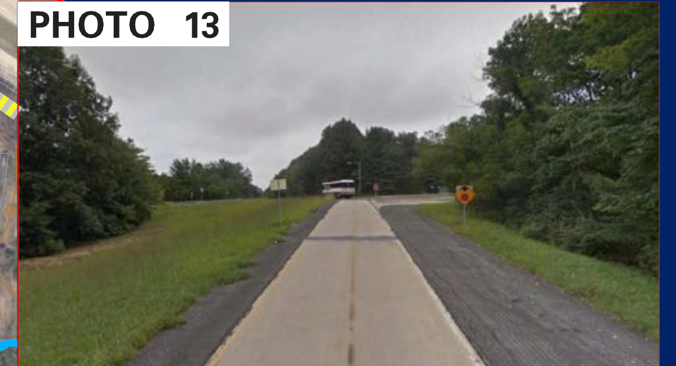
INTERSECTION OF 202 OFF RAMP 2 AND EASTON ROAD/MAIN STREET
