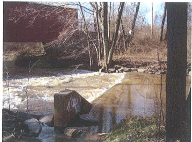
Pine Run Creek near the existing covered bridge
