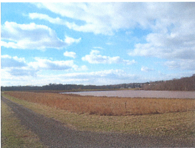
View of existing maintenance road
