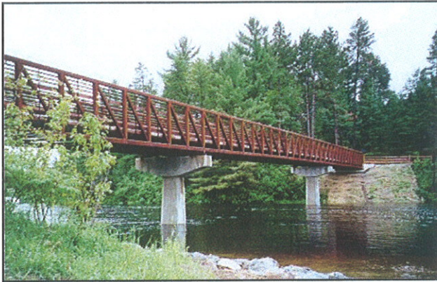
Example of Independent Trail Bridge
