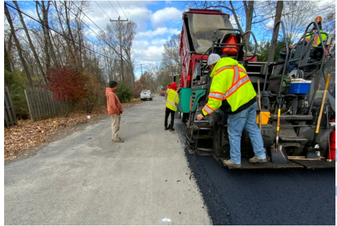
Paving Machine Laying Pavement
