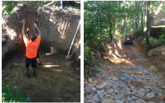
Drainage Project on Springs Dr.
