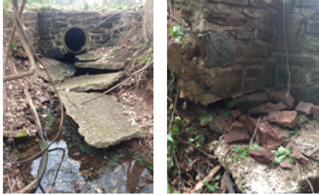
Endwall and outfall stabilization on Pebble Crest Dr.
