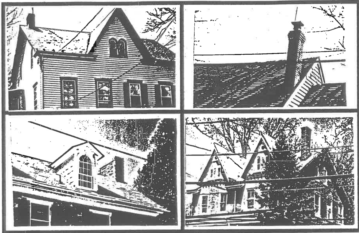
Photos 6.23 - 6.26 Gables, Dormers, Gutters and Chimneys
