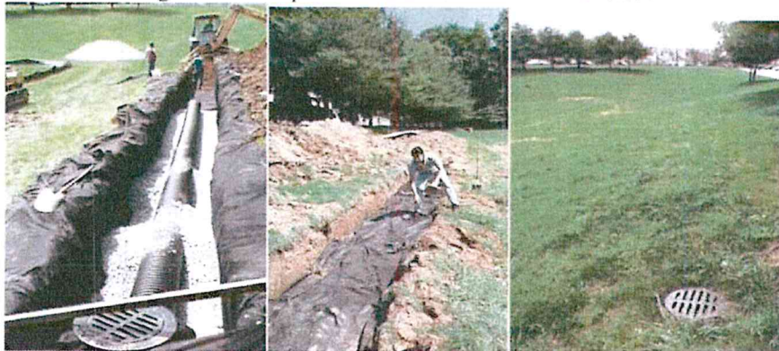
Figure 4: Example of Infiltration Trench Installation
