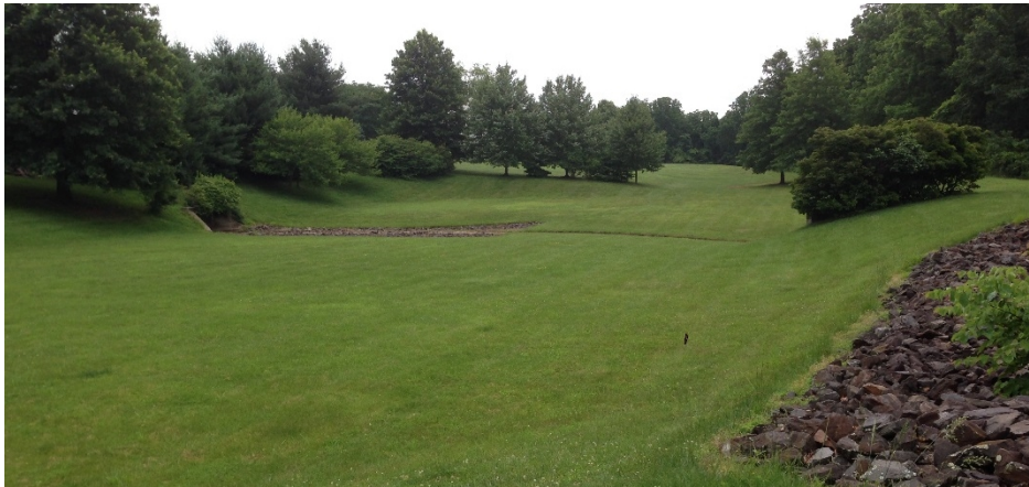
Photo 4 - Proposed BMP-B: Ridings at Covered Bridge BMP Retrofits
