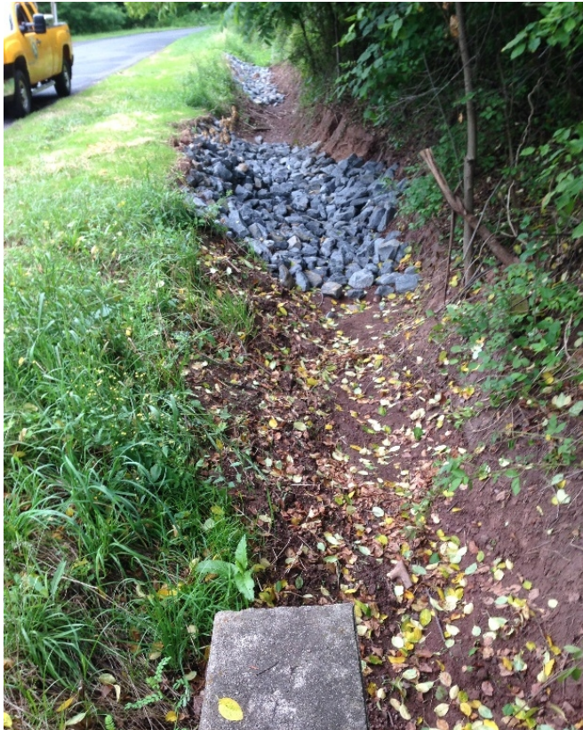
Photo 7 - Proposed BMP-C: Pine Run Road Stream Restoration
