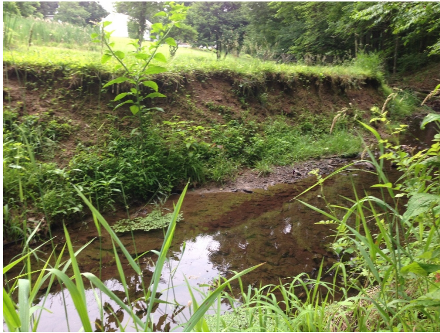
Photo 1 - Proposed BMP-A: UNT Neshaminy Creek Stream Restoration
