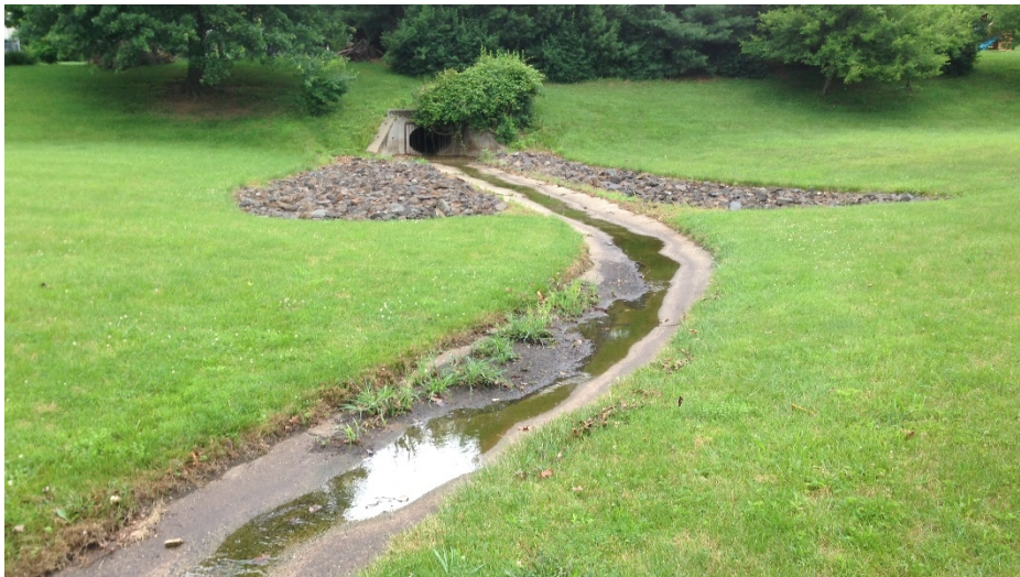
Photo 5 - Proposed BMP-B: Ridings at Covered Bridge BMP Retrofits
