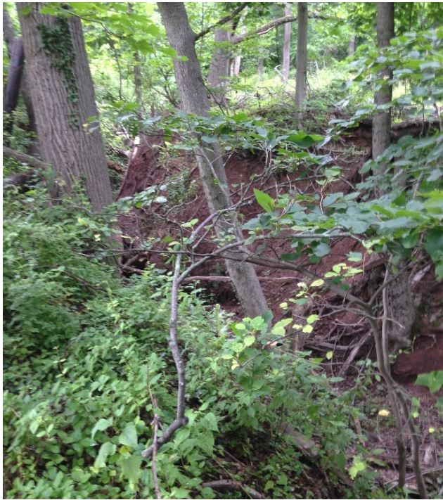
Photo 6 - Proposed BMP-C: Pine Run Road Stream Restoration
