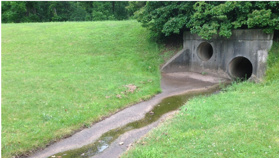
Photo 3 - Proposed BMP-B: Ridings at Covered Bridge BMP Retrofits
