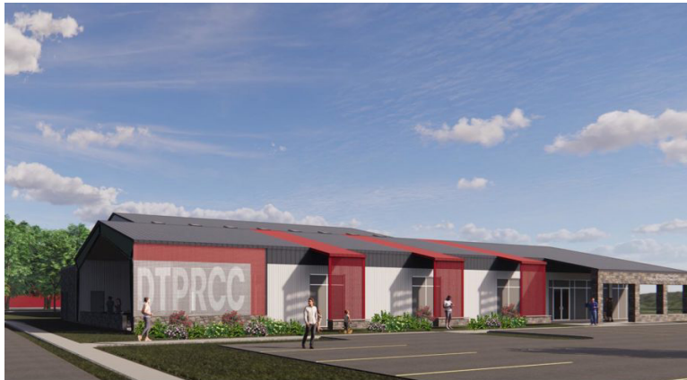
DOYLESTOWN TOWNSHIP PARKS & RECREATION COMMUNITY CENTER VIEW OF PORCH AND ENTRY
