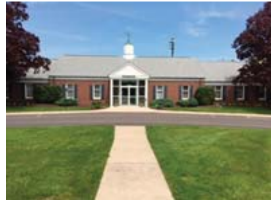
Township Building Main Entrance
